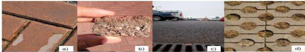
Figure 1. (a) Impermeable concrete interlocking pavers; (b) porous concrete; (c) porous asphalt; (d) grass-filled grid pavers.
